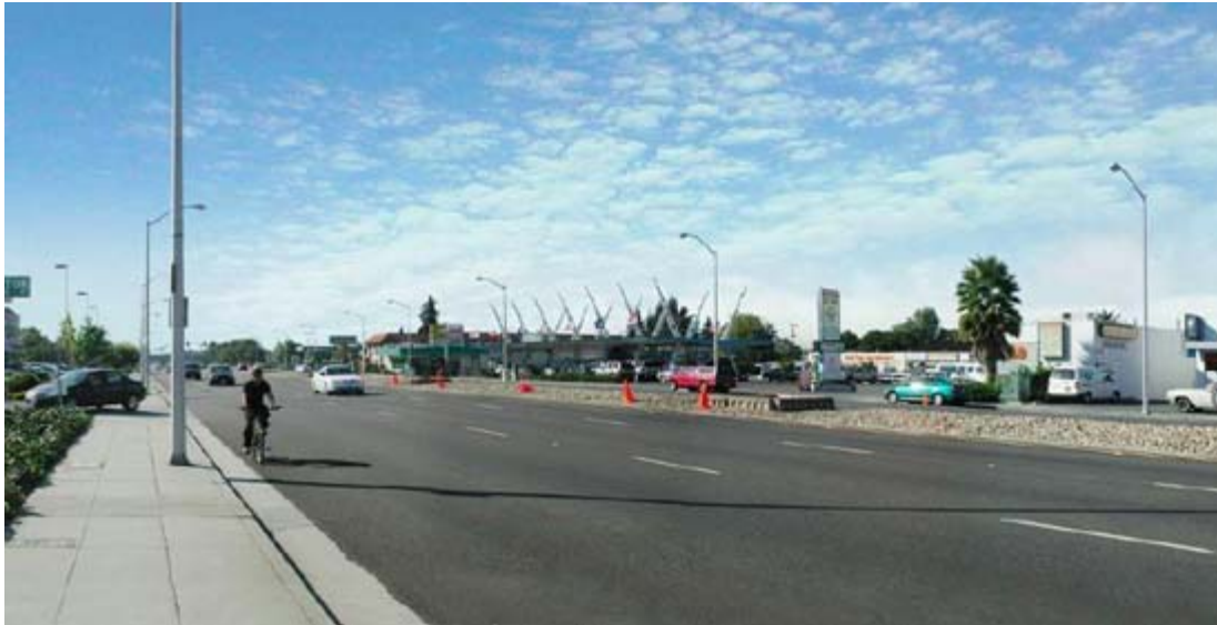
BRT corridor currently. Photo: San Jose DOT.
